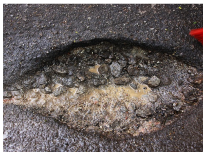
Brush out debris
