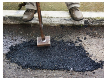
Tamp down. Ready for trafficking
